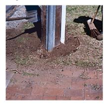
Finally check that the top of the Ausplast is in contact with the pole around the full circumference. Backfill excavated material applying foot compaction to ensure the paste is pressed in intimate contact with the pole. The finished natural surface must be re-established with top of the Ausplast 50 mm. below and otherwise to the pole owner's instructions.
